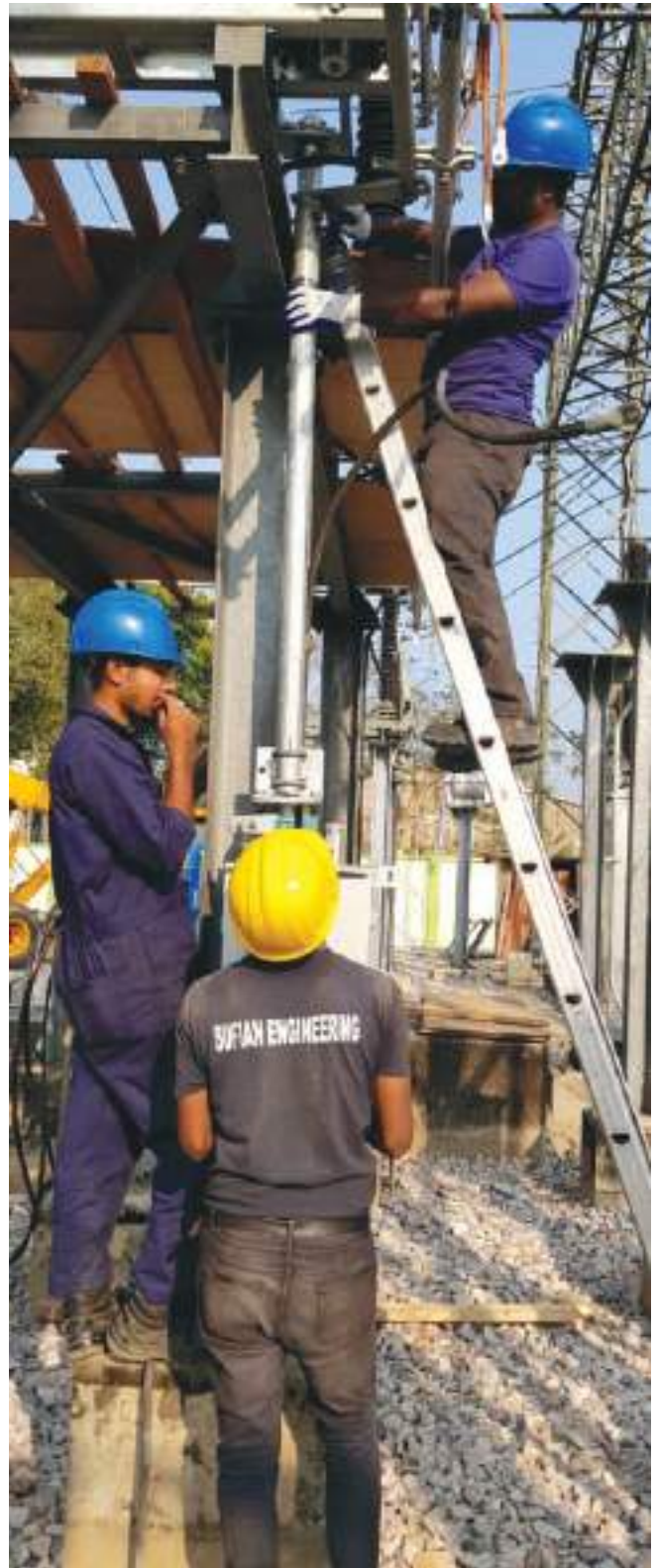
Substation work at Karnafull Hydropower Station, Kaptai
