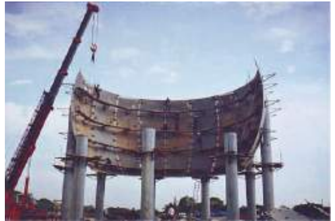
The Construction of two LPG storage spheres of 2500 M 3 each as per French standard Codap 95 in Kumira, Chittagong
