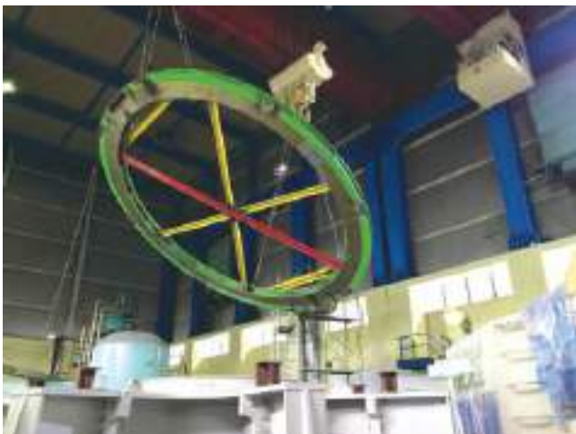
Turbine over hauling
