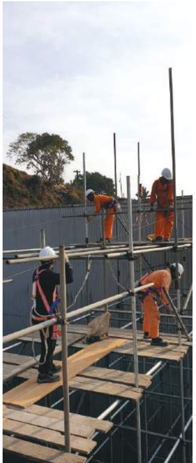
Karnafuli Hydropower Station, Kaptai
