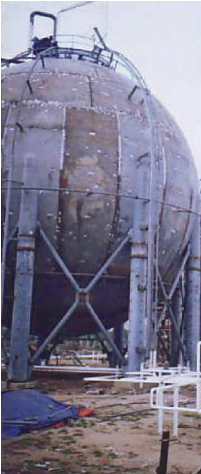
The Construction of two LPG storage spheres of 2500 M 3 each as per French standard Codap 95 in Kumira, Chittagong
