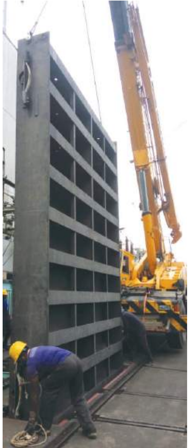
Bulk head gate maintenance
